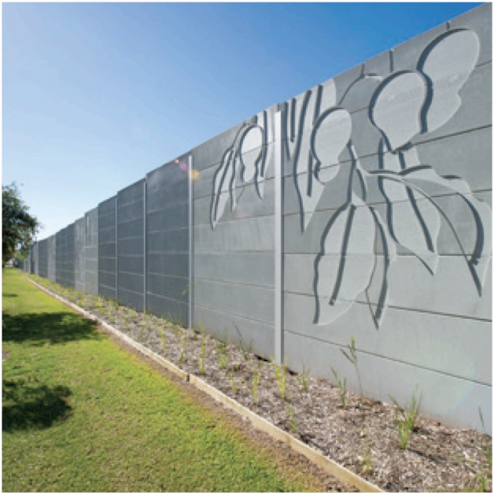
Hebel or similar aerated concrete panels with rebate detailing and paint finish
